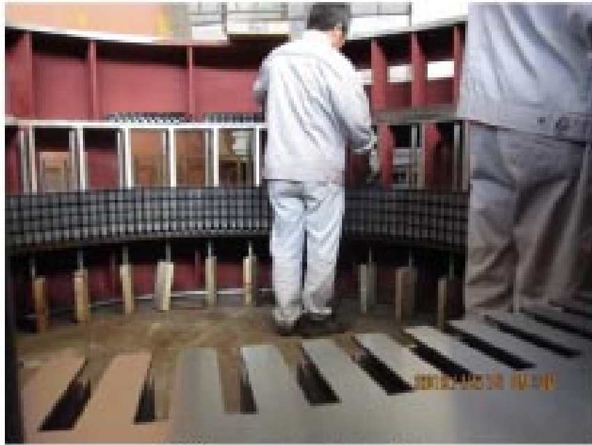
Fitting generator stator plates
